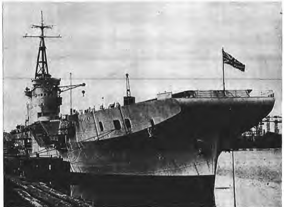
This photo of HMS Perseus shows the forward part of the raised flight deck which was built to meet the requirements of the revolutionary steam-operated aircraft catapult. The catapult reduces the need for a carrier to steam into the wind to fly off its aircraft and enables it to launch new and heavier types of planes. (United Kingdom Information Office Photo).
