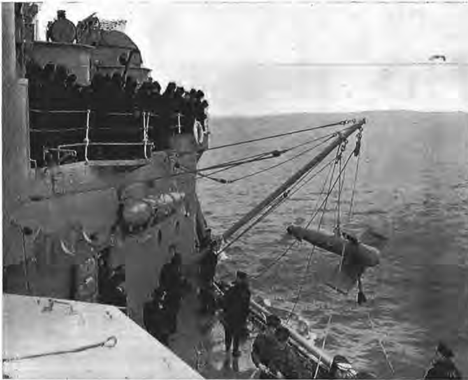
Rigging and streaming of paravanes was one of the many evolutions carried out in the Quebec as the cruiser steamed from West Coast to East. (QB-12).
