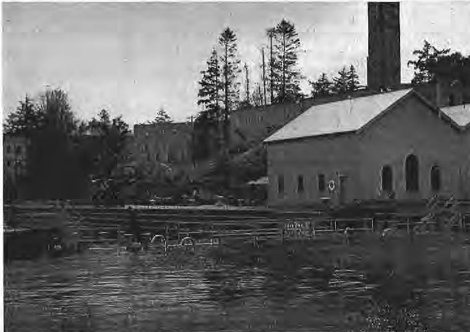
The end of November brought some of the highest tides seen in Victoria in many years. Shown here is the water topping the gates of the naval drydock at Esquimalt. (E-17126).
