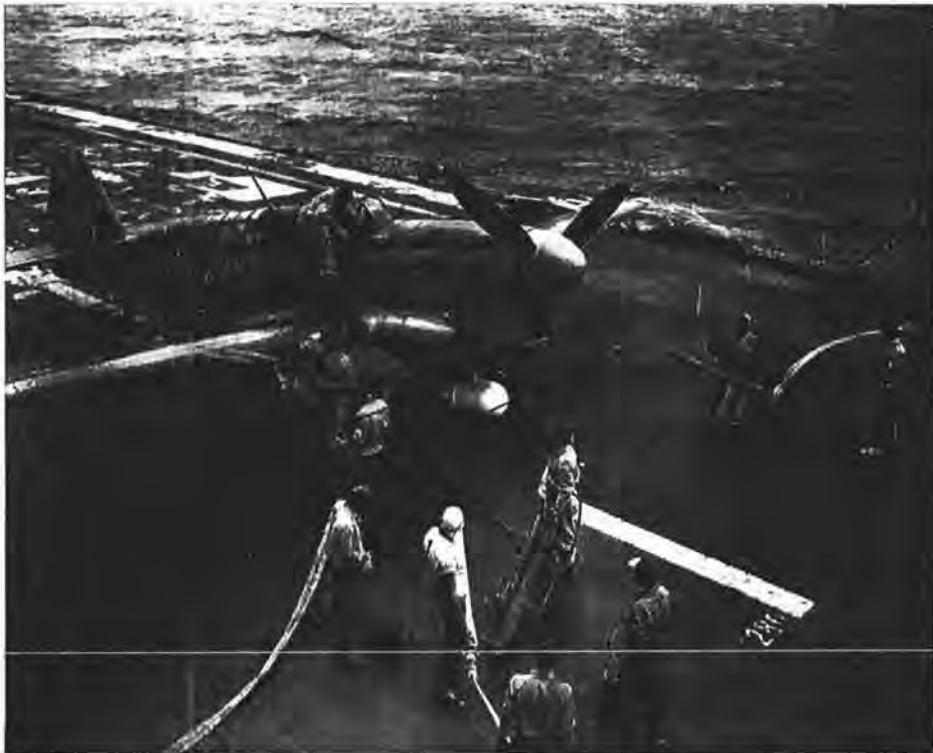
The "Magnificent's" flight deck fire-fighting party carries out rescue drill in a simulated barrier crash. The rescuers wear asbestos suits that enable them to wade into the midst of fires. Other members of the team stand by with CO 2 and foam apparatus. (Mag-1548).
